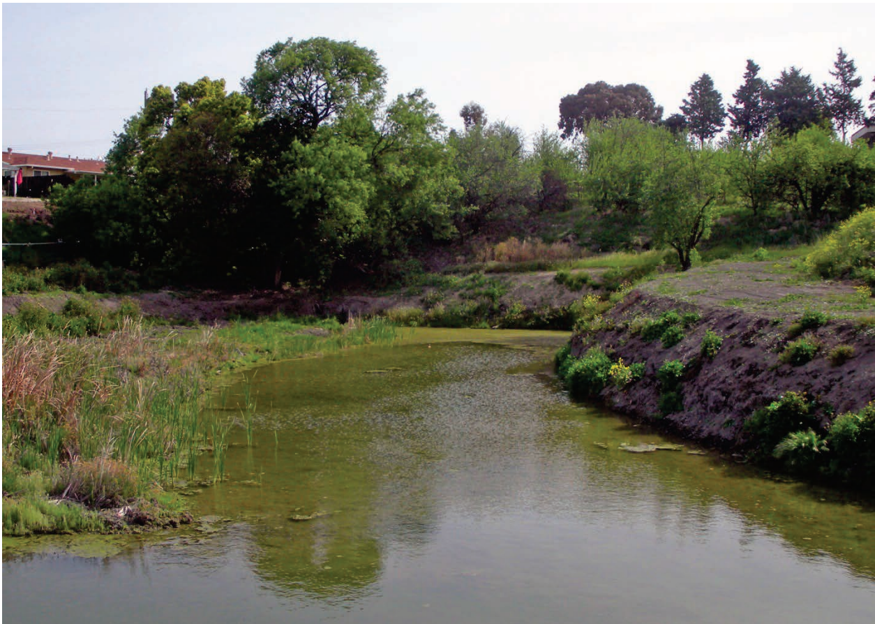
Figure C-11. Sludge Pond Upgrades
