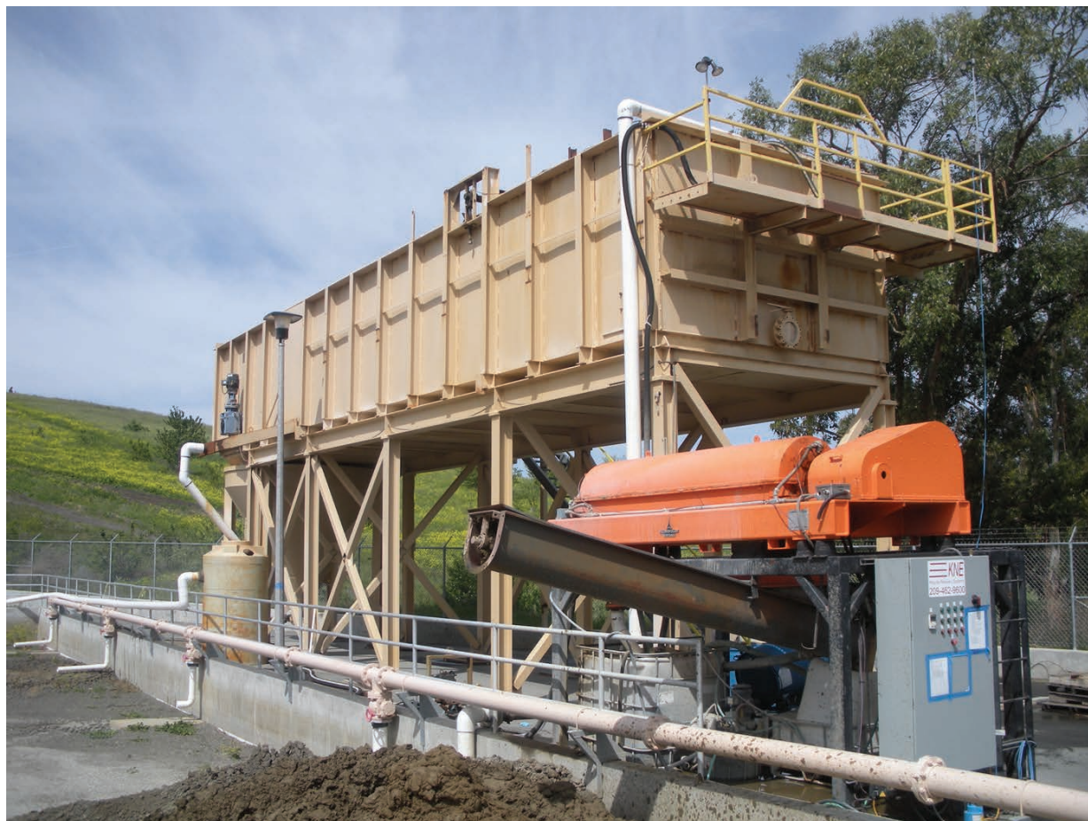
Figure C-6. Sludge Handling Improvements
