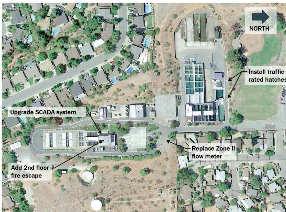
Figure C-4b. Some WTP Upgrades
