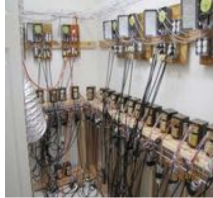
Residential Electrical Rewiring source: Chief Marc Vasquez.
