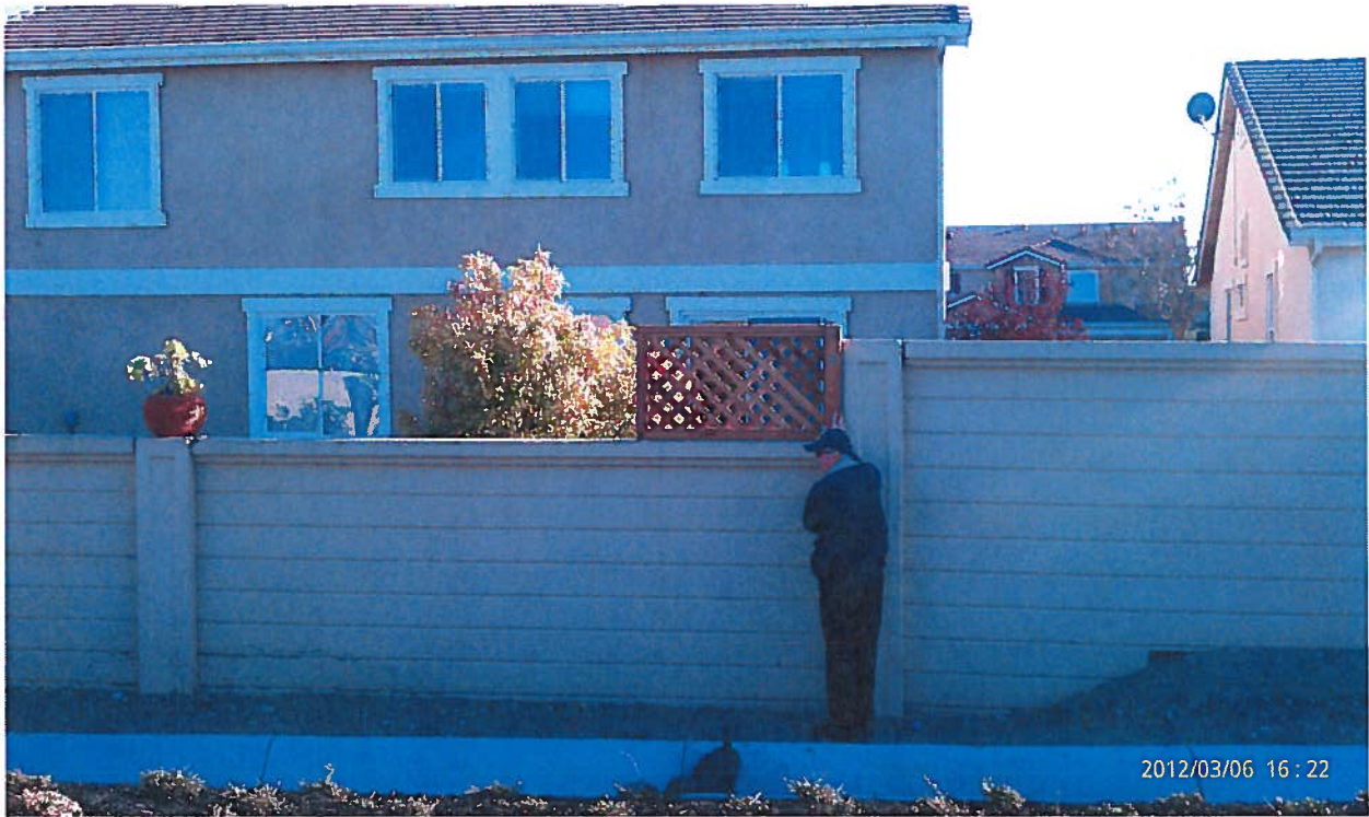
4625 Menona Court: 2'-high lattice sample on rear wall.
