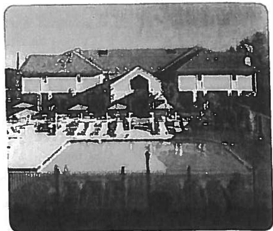
Figure 3.2.23 A swimming pool shielded from the public street provides a private amenity
