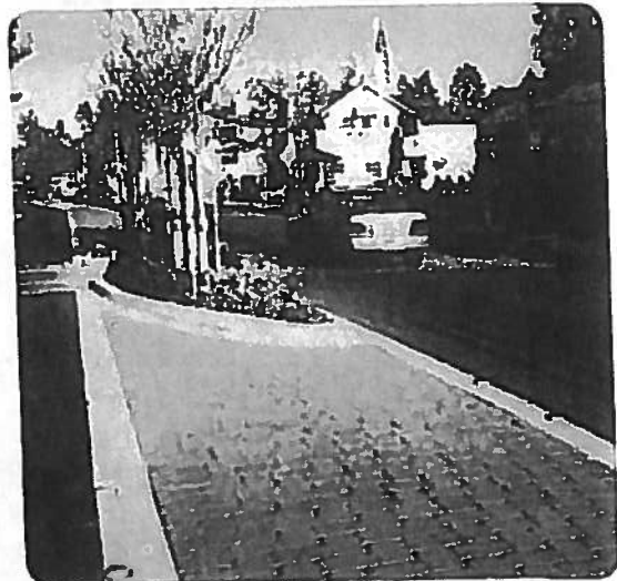
Figure 8.3.18 The pavers in this median contrast with the asphalt in the driving lanes
