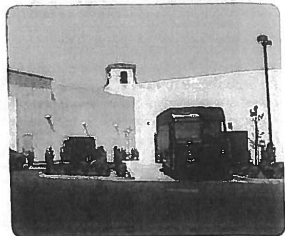
Figure 4.6.1 A loading facility that is screened from public view by placement in the rear of the building
