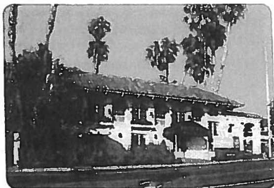
Figure 3.2.22 A motel with the building and driveway approach facing the street
