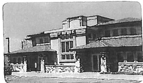
Figure 4.2.1 Selection of appropriate architectural style and quality of design add to the character of the neighborhood
