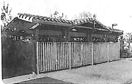
Figure 3.1.14 Screening of trash enclosures through metal doors and masonry walls
