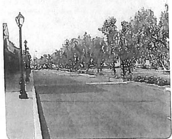
Figure 3.1.24 A major access drive with no parking
