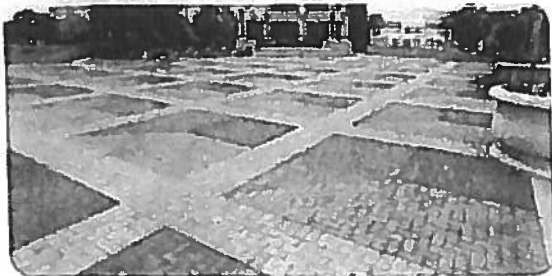
Figure 4.3.8 Permeable paving materials can be visually interesting
