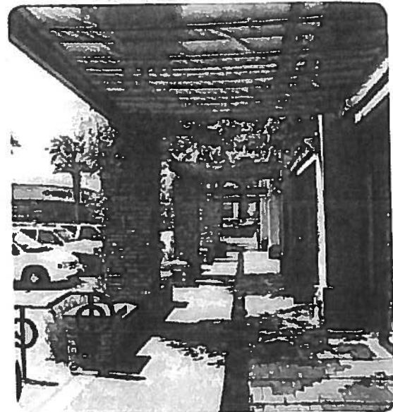
Figure 3.2.5 A canopy provides protection against sun and rain
