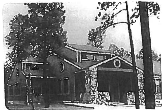
Figure 3.2.29 An interesting office building design complements the neighborhood character
