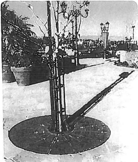
Figure 3.1.9 A tree grate and guard
