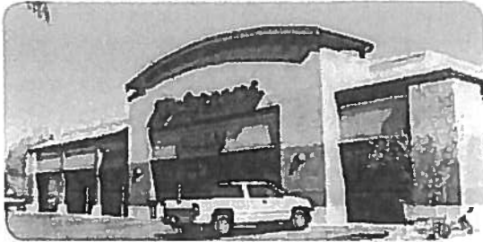
Figure 3.1.15 A structure that uses canopies, columns and recesses to provide vertical and horizontal articulation
