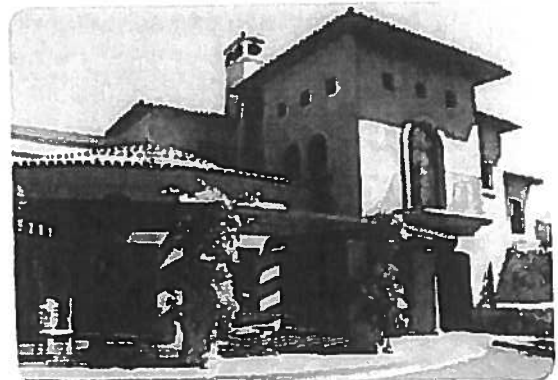
Figure 3.2.31 An office building provides functional vertical and horizontal wall plane offsets
