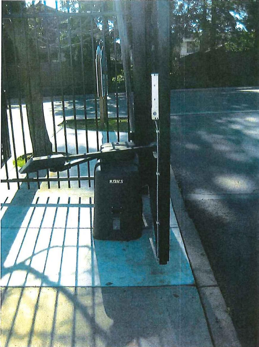
Figure 9: South access gate to the Contra Loma Apartments Complex. Photo is looking southerly at the right swing gate and gate mechanism. The proposed X2 Swing gate system to be utilized at the Contra Loma Estates project eliminates the exterior motor and gate arm. All components are contained within the fixed gate column. See figures 13, 14 & 15 which follow.
